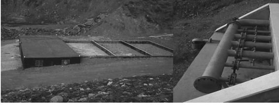
Fig. 4: Chemical-physical (CP) plant of the leachate, sludge drying beds and gas collection system (Bilgin et al. 2008, Erdin 1999, 2001, 2008)
