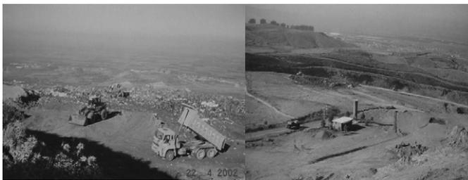
Fig. 3: Tipping, Spreading and Compression of the waste on the landfill surface and collection and incineration of the landfill gas formed at the first section of the landfill (Bilgin et al. 2008, Erdin 1999, 2001, 2008)
